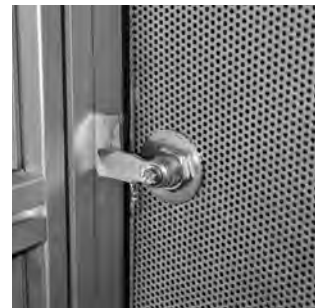
panel firmly bolted together
